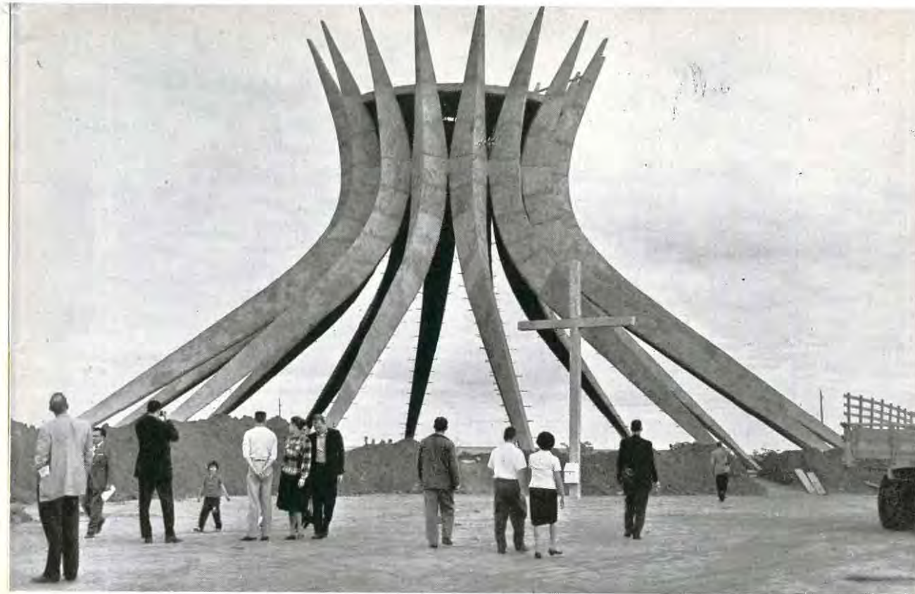
A Catedral em fase de acabamento, pronta para receber as chapas de vidros que a revestirão. The Cathedral, in its final stages, awaiting to be covered by large sheets of refractory glass. La Cathédrale, en phase d'achèvement, prête à être recouverte de larges panneaux de vitre.
